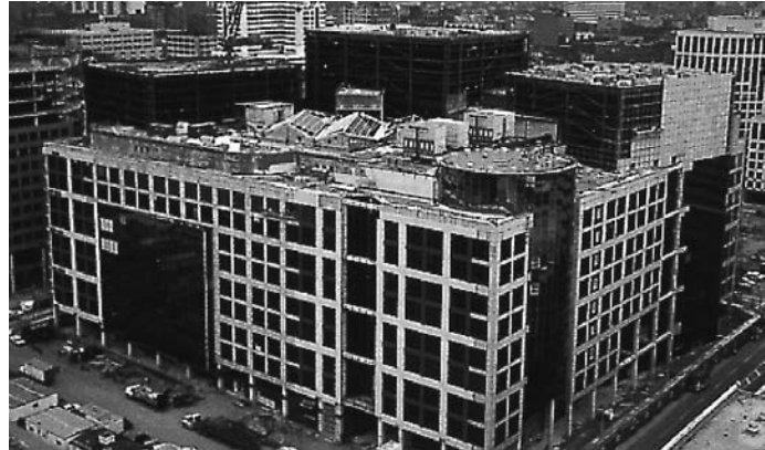
Photo of CBC project during construction. Note the three large roof top studios still exposed (the largest is approx. 70 feet high).
