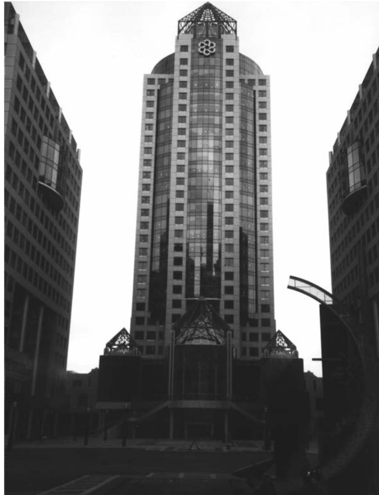
Vibro-Acoustics supplies silencing packages for on-floor air handling units.
