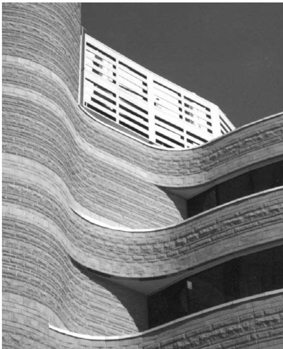
View #1: Looking up through the acoustical louver air passage.
