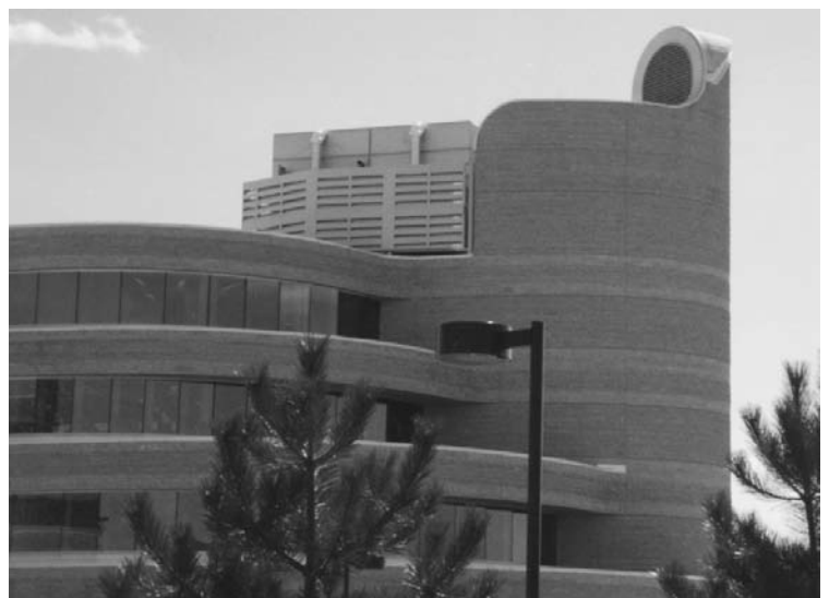
View #2: Acoustical louvers block cooling tower air intake's line of sight.
