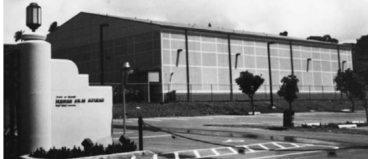
Special silencing designed and supplied for TV production facility project.
